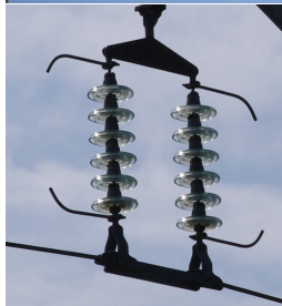
a module of cap and pin insulator
